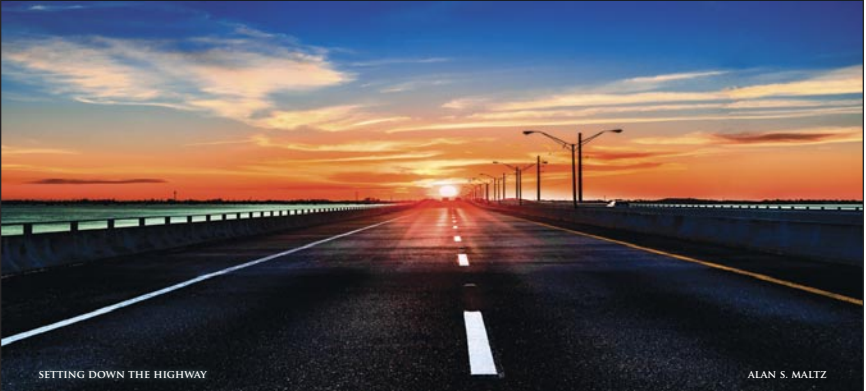
SETTING DOWN THE HIGHWAY
